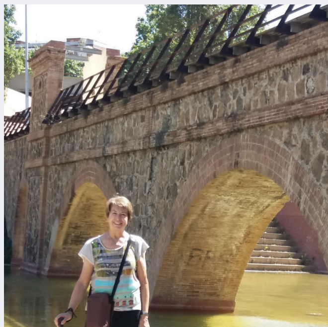
Dosrius aqueduct, built in XIX Century to bring water from a northern area of Barcelona
